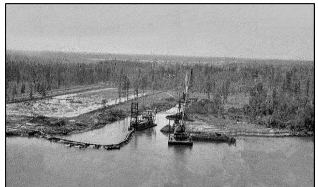
The berth for Battleship North Carolina is dredged in anticipation of an October 1961 Wilmington arrival.
