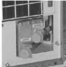
On the upper section, 2 air bleed valves ensure the correct operation of the hydraulic coil.
