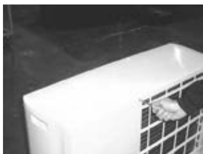
Remove the central screw (at the back)
