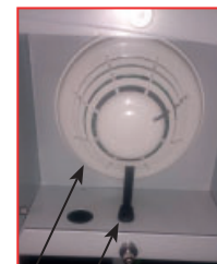
Air inlet tube Smoke detecting probe
