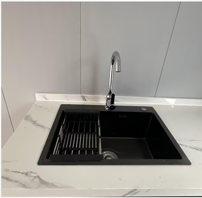
1 sinks +drain basket
