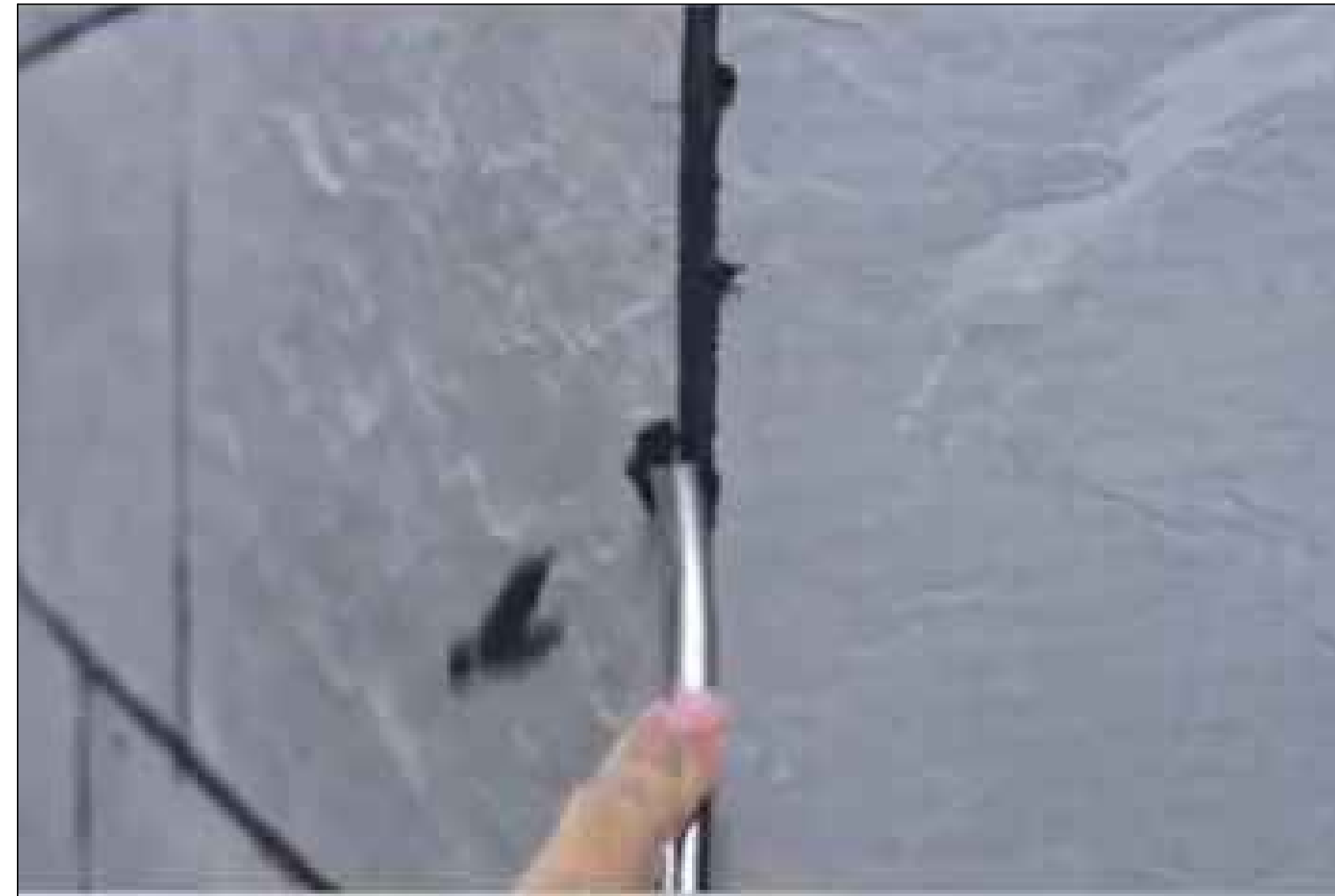
SMOOTHENING OF GROUTS AT EDGE
