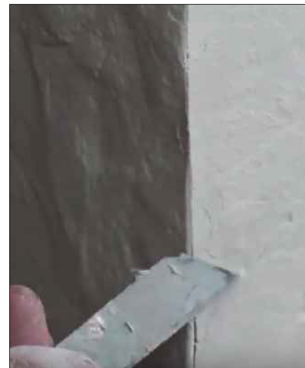
GROUTING AT THE JOINT
