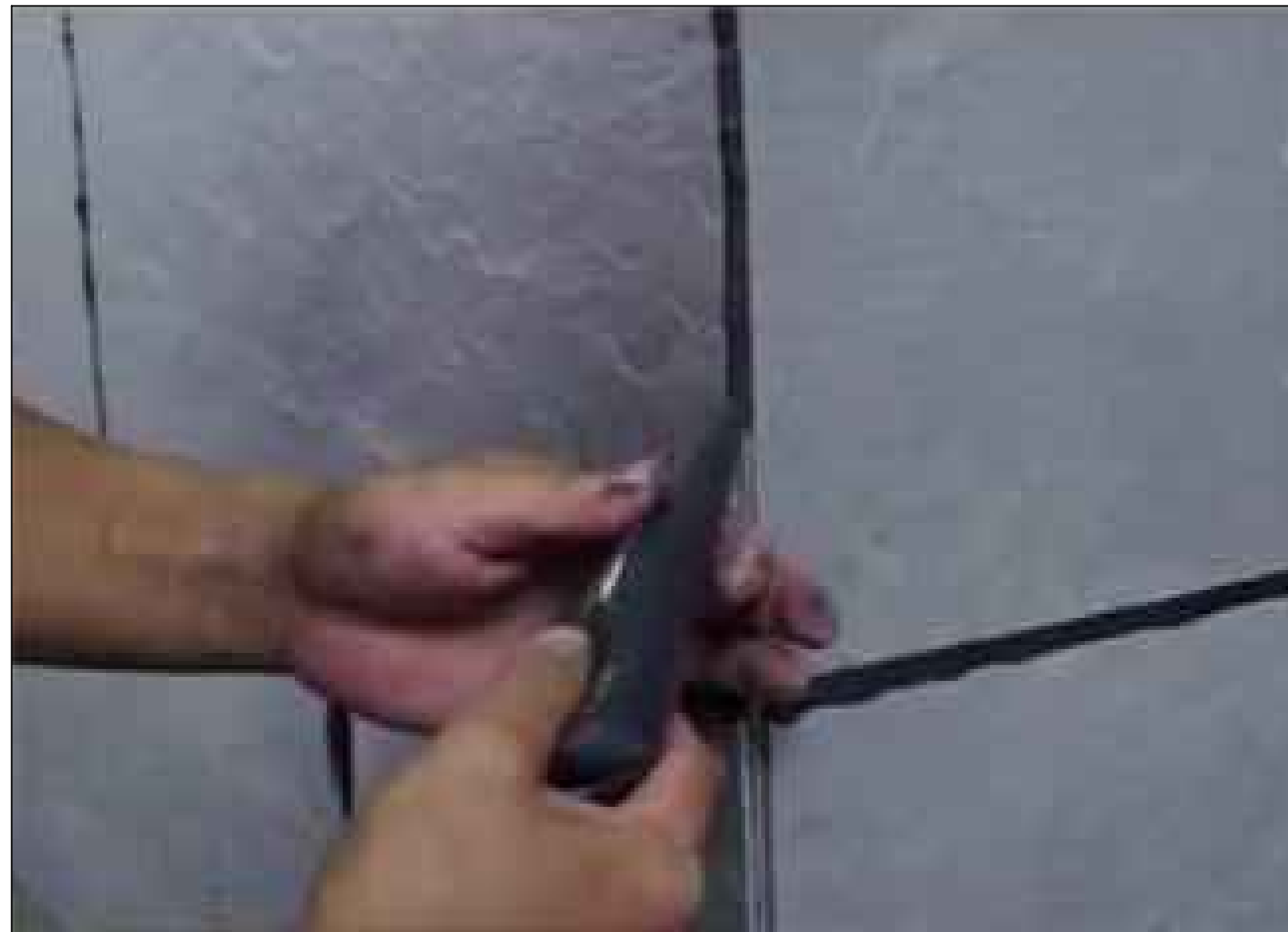
GROUTING AT EDGE
