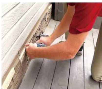
4. Lay the panels down to up, left to right, fix the panels with screws on the joints, 从左至右, 由下至上安装, 用螺丝固定
