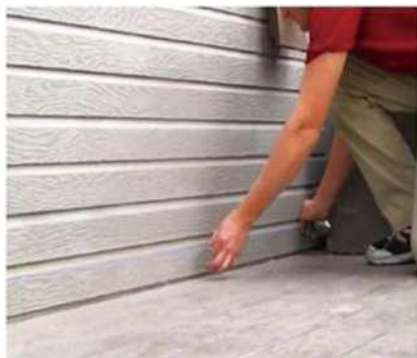
1. Level and color up the wall horizontally. 在墙底拉水平线
