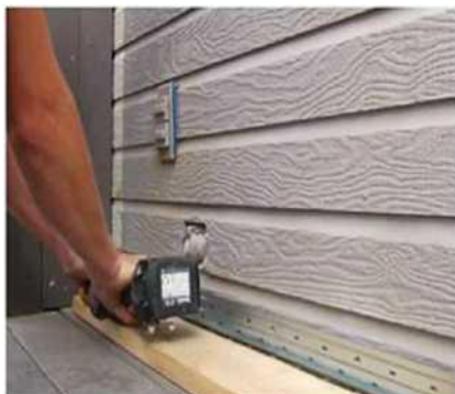
2. Put the starter strip on the bottom of the wall. 在墙底装水平条
