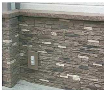
6. Keep on installing the panel & corners and top lines, 完成安装墙板、转角及收边
