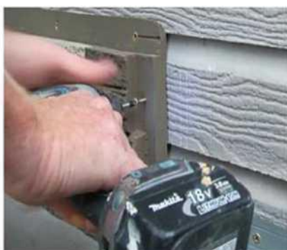
Drill the screw through the center of the joints to the wall. 打螺丝的时候在舌边的中间打入
