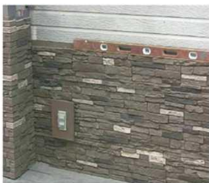
5. Check if the panels are horizontal with a level during installation, 安装过程中用水平尺测试是否平整
