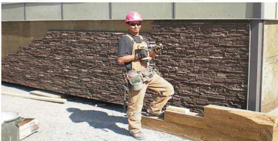
Drill the screw through the center of the joints to the wall. 打螺丝的时候在舌边的中间打入
