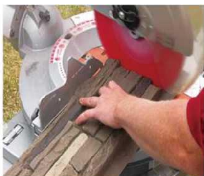
Cut the panel with a saw if necessary. 用手锯或电锯切割
