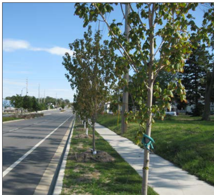
Lawn strips should be at least large enough to accommodate growth and root expansion to prevent sidewalk and curb damage.
