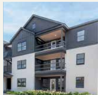
Emerson at Commonwealth
