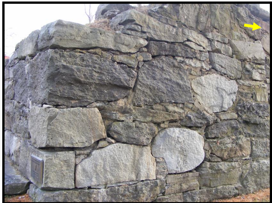
G.C.A. 6 Westerly face of the Gill cable anchor, about 8 feet high on left edge, shows the diverse rock types. There are three rounded granite boulders, plus angular quarried local sedimentary rocks. A
