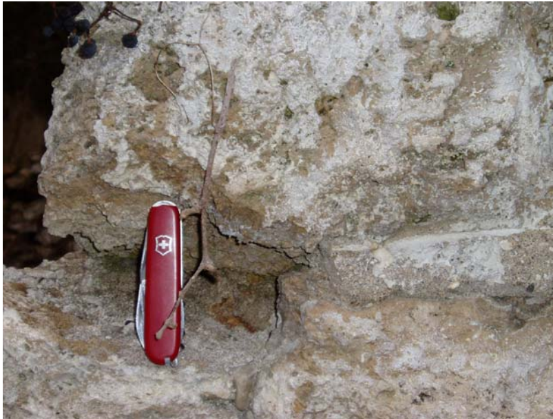
Photo 1. Detail of tufa porous tufa stone from block used in the foundation of a small barn near the tufa mound site. The pores are mostly the result of the precipitation of limestone ( \text{CaCO}_3 ) around vegetative matter which subsequently decomposes.
