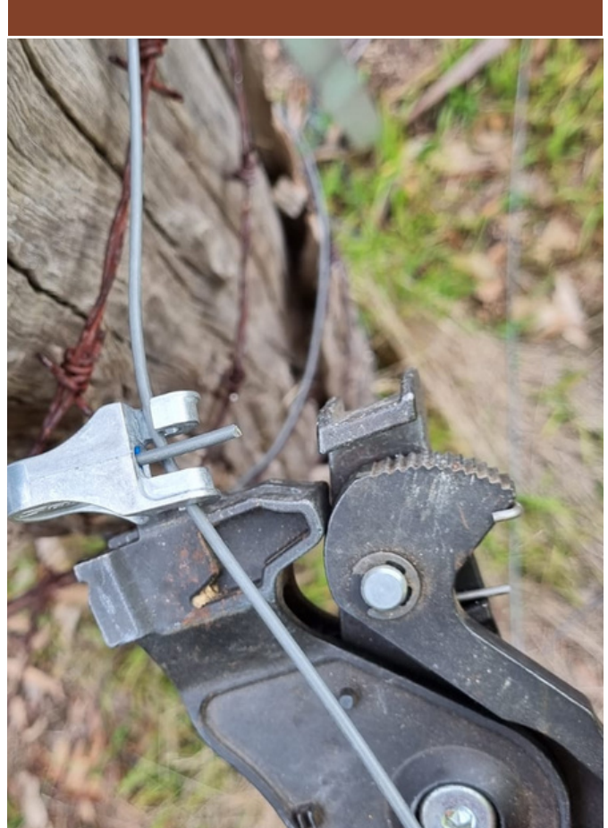
Above: Tail wire trimmed too short
