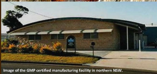
Image of the GMP certified manufacturing facility in northern NSW.
