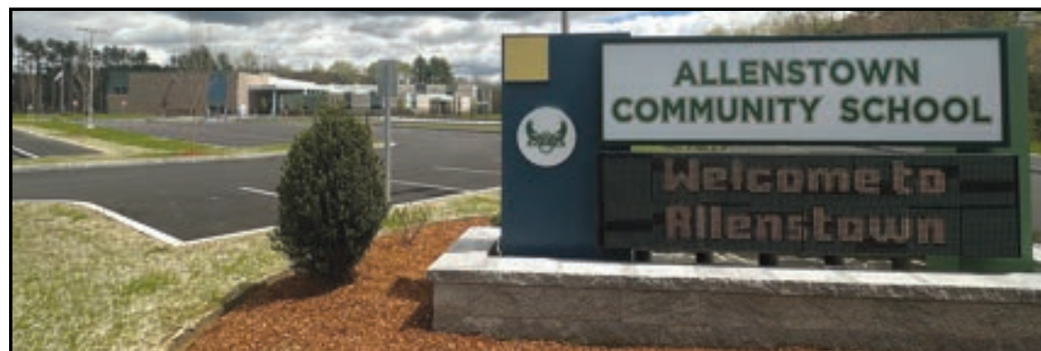
The new Allenstown Community School. (Tony LaCasse Photo)
