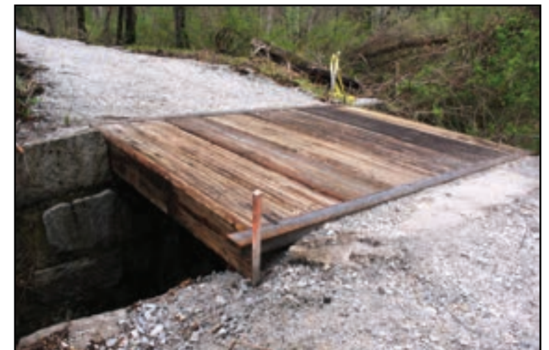
Old bridge. (Michael Frascinella Photo)
