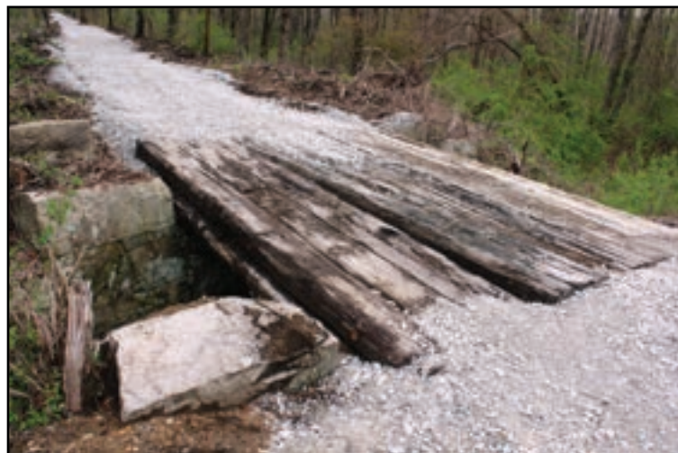
Old bridge. (Michael Frascinella Photo)
