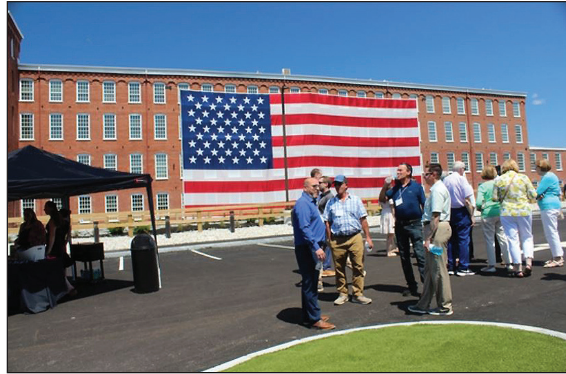
READY FOR RESIDENTS - 25 Canal Residential Lofts was officially opened with a dedication on July 20. The "Great Flag" displayed on the building is a 90x50-foot replica of the flag produced by the Amoskeag Manufacturing Company in 1914 and displayed by mill workers in the Manchester millyard. The Great Flag went missing after an appearance in a New York City parade in 1916. Brady-Sullivan purchased the current flag in 2012, and uses it for all their grand openings. (Courtesy photo)
