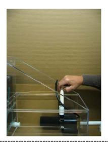
Slip threaded Tee (II) over 31/4" length section of 1/2" PVC Pipe (II)
