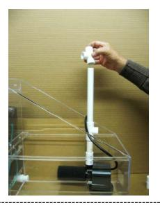
Insert  $1\frac{1}{2}$ " length section of  $\frac{1}{2}$ " PVC Pipe (V) into  $\frac{1}{2}$ " Tee (V)
