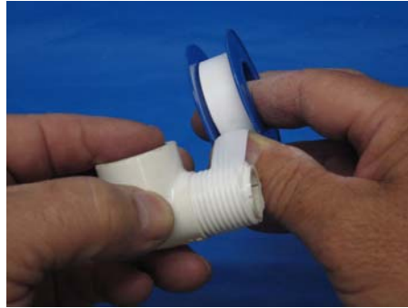
(2) Apply Teflon tape to threads.
