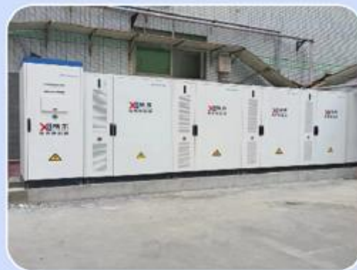
Changan Chensong Station
