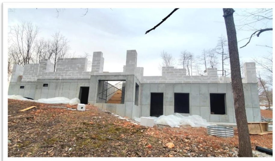
Figure 5: Concrete Foundation w/AAC Block, Bentonville Arkansas
