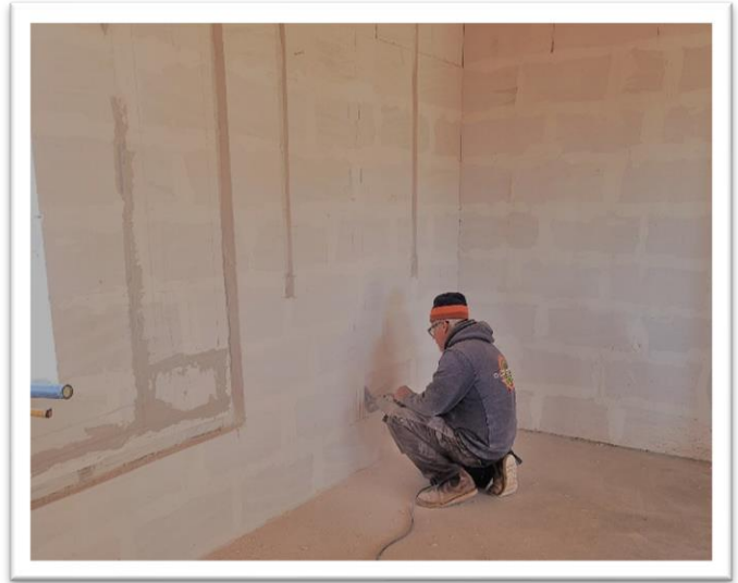
Figure 2: Worker routing out Rough-in Electrical and Plumbing
