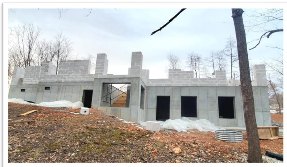
Figure 5: Concrete Foundation with AAC Block, Bentonville Arkansas
