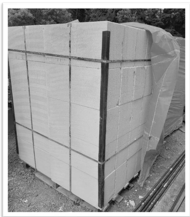
Figure 6: One Pallet Contains 60 Blocks of 12x8x24.
