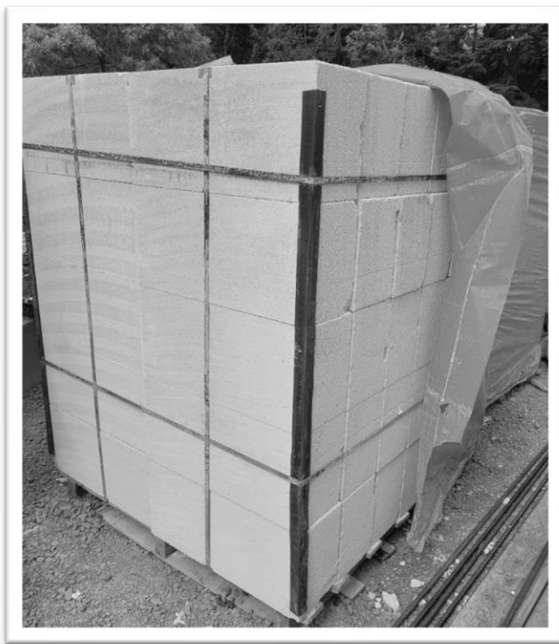
Figure 7: One Pallet Contains 60 Blocks of 12x8x24.
