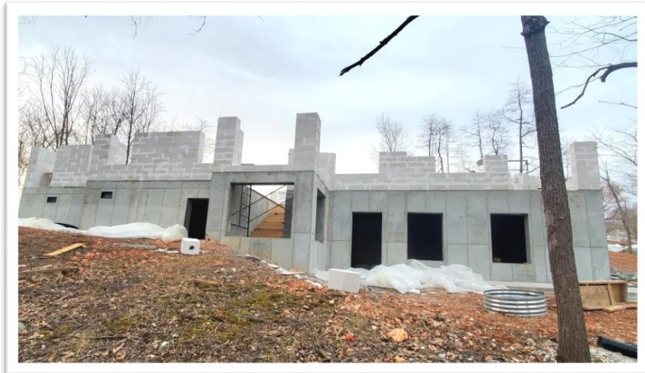
Figure 6: Concrete Foundation with AAC Block, Bentonville Arkansas
