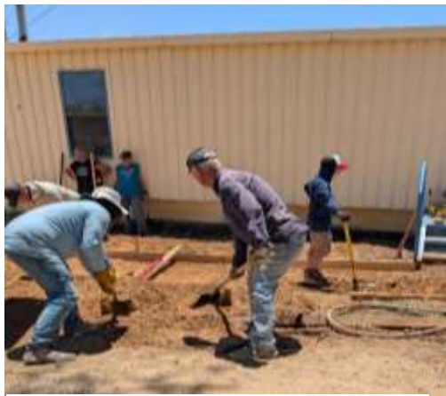
Building sidewalks at St. Joseph Mission School
