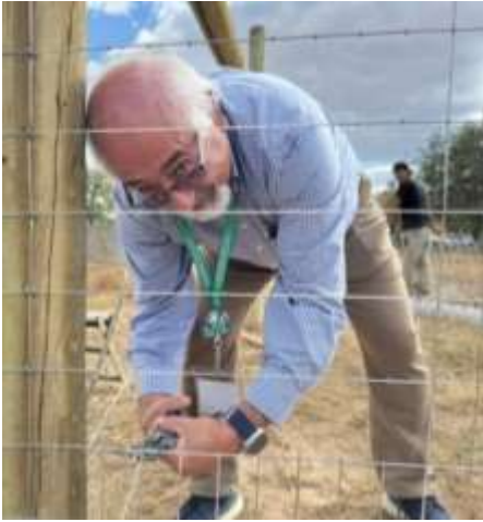
Antonio working on the fence
