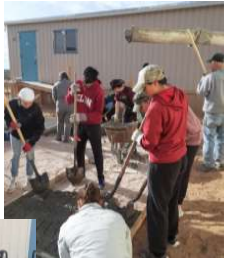
Reuben and students during the concrete pour
