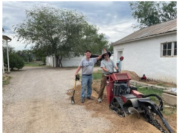
Bruce enjoyed using the big toy, a trencher, donated by Mountain States Constructors.
