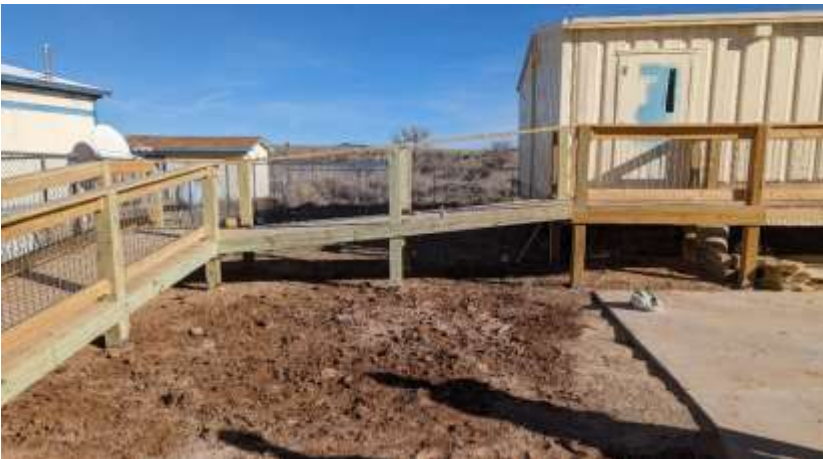
Part of the almost- finished deck and ramp
