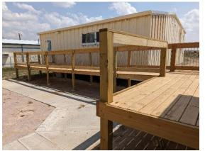
the month of July, they built a ramp and decking to and between the portable classrooms, providing handicap access to the classrooms. During August, they constructed a
