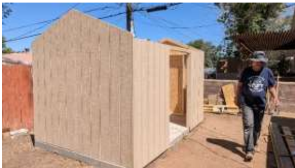
Bob with the almost-finished shed
