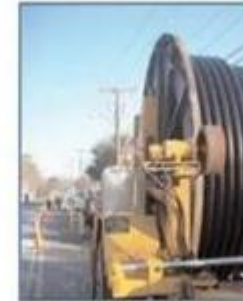
■ Pull and splice cable
