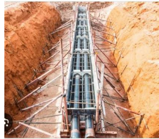
TenneT Energy - Netherlands, 2015, 525kV HVDC cable, 2GW
