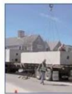
■ Installation of manholes
