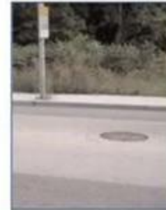
■ Backfill trench and install temporary concrete
