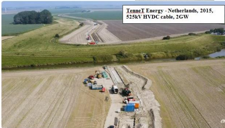
TenneT: Laying of direct current underground cables (HVDC)
