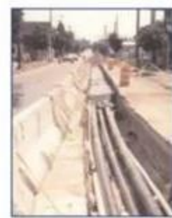
■ Lay conduit and encase in concrete
