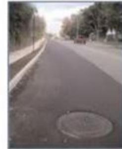
■ Final treatment with new asphalt
