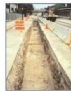
■ Mark location of line and dig trench
