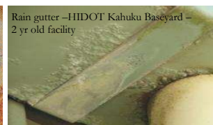
Late Stage 2 corrosion conditions.
