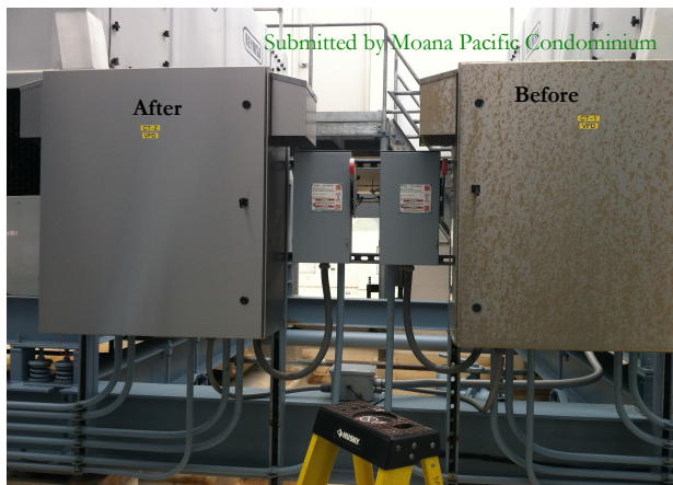
Stage 1 - Earliest signs of corrosion.
