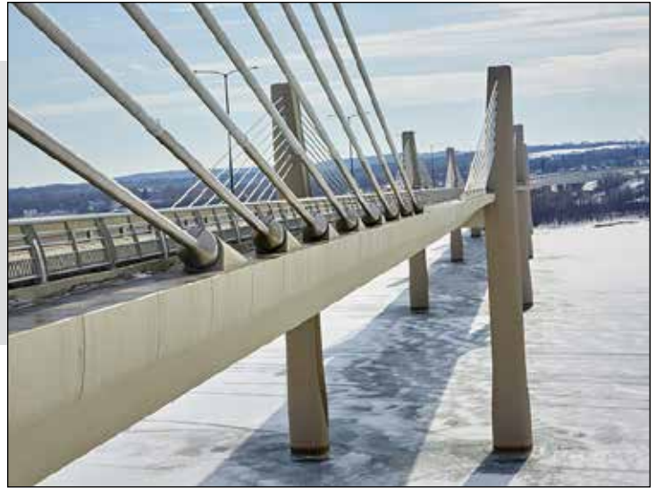
St. Croix River Crossing
