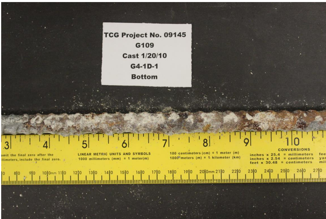
Figure 9 – Top Bar from Control Beam, showing the bottom surface
