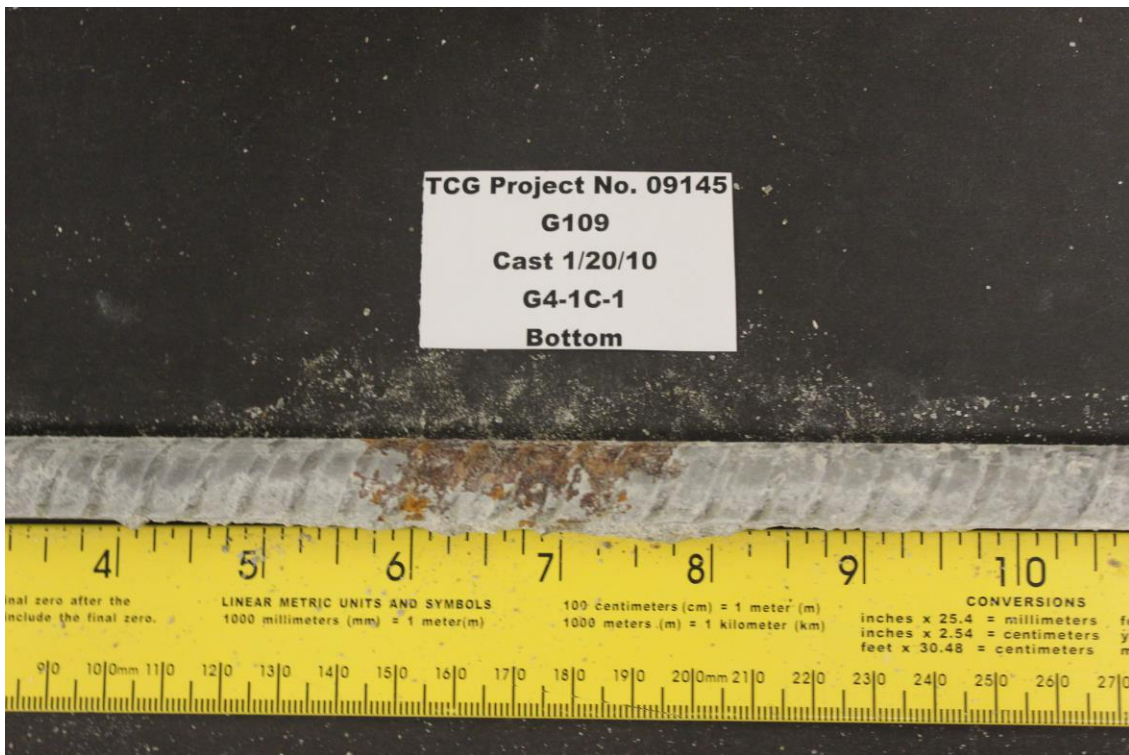
Figure 7 – Top Bar from Control Beam, showing the bottom surface
