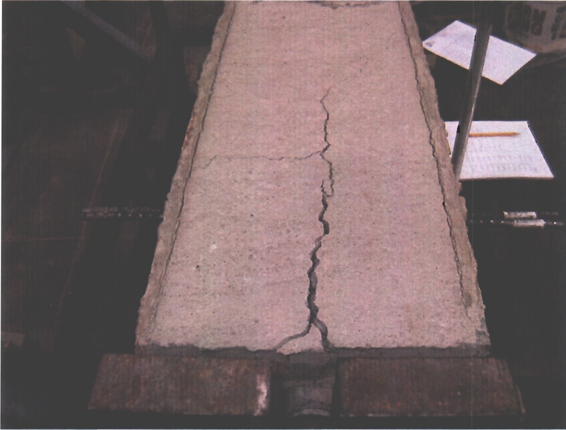
Photo 3: Typical failure of specimens
