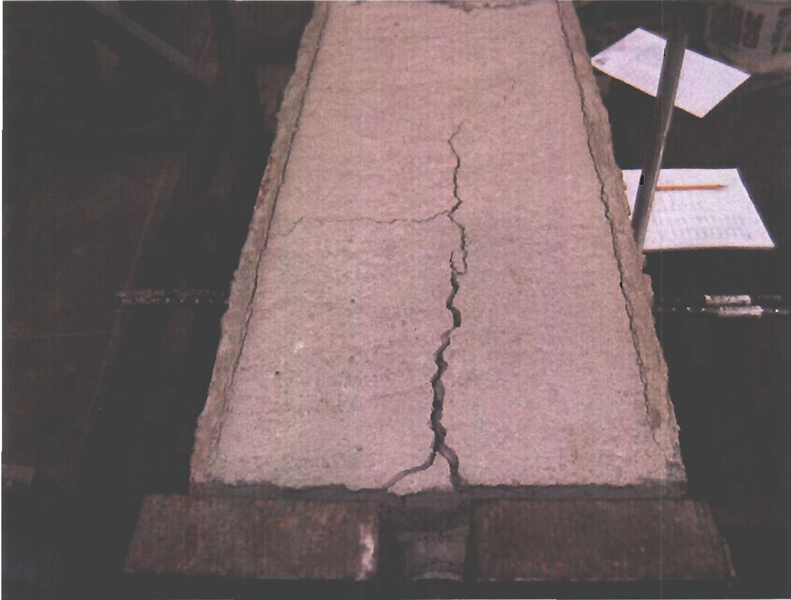
Photo 3: Typical failure of specimens
