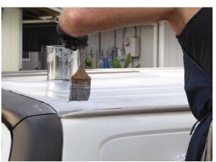
Step 9 – Applying  $\mathbf{1}^{st}$  coat - Cortec VpCI-396 Moisture Cure Urethane\*
