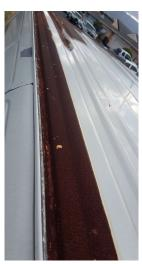
Step 5, Step 6 and Step 7 – Prepping surface to tight rust
