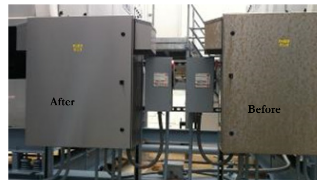
Moana Pacific Roof Top Stainless Steel Control Cabinets
