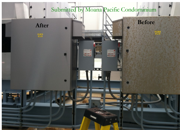
Stage 1 - Earliest signs of corrosion.
