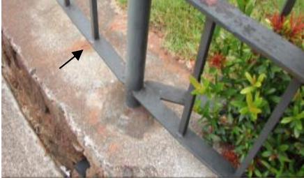
Maintained welds annually with CarWell CP90
