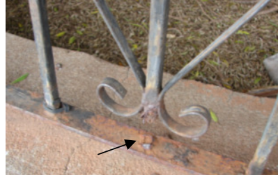
Unmaintained –destroyed by the effects of corrosion. Preventable with annual application of CarWell CP90.
