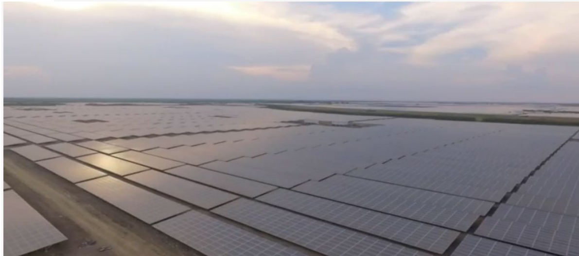
Kamuthi Solar Power Project – 648MW – India
