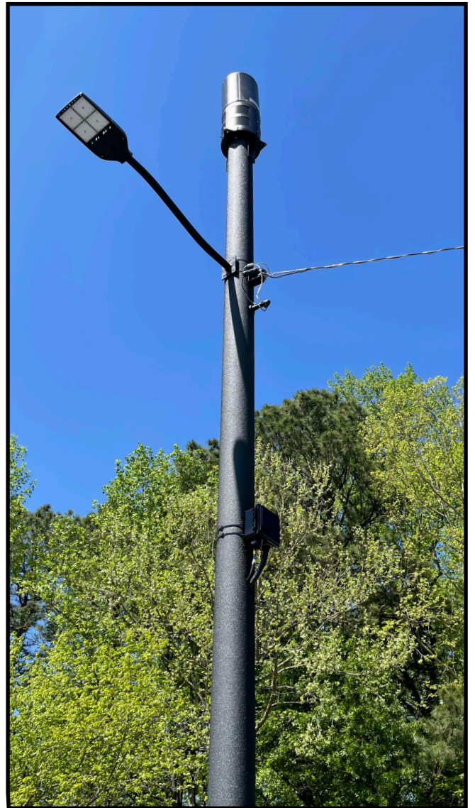
Left, final site following tower installation. Right, detailed view of disconnect, lighting fixture and RF equipment.
