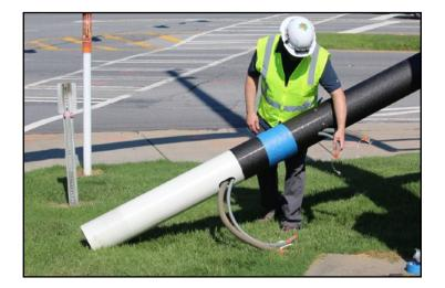
EasyStreet Systems Field Engineer Mason Kelley inspecting the pole prior to install. Custom access port made for conduit lines was cut using simple hand tools. White uncoated portion of the pole goes into the ground for direct bury system. Blue tape temporarily applied to keep rapid-set foundation from adhering to the pole surface.
