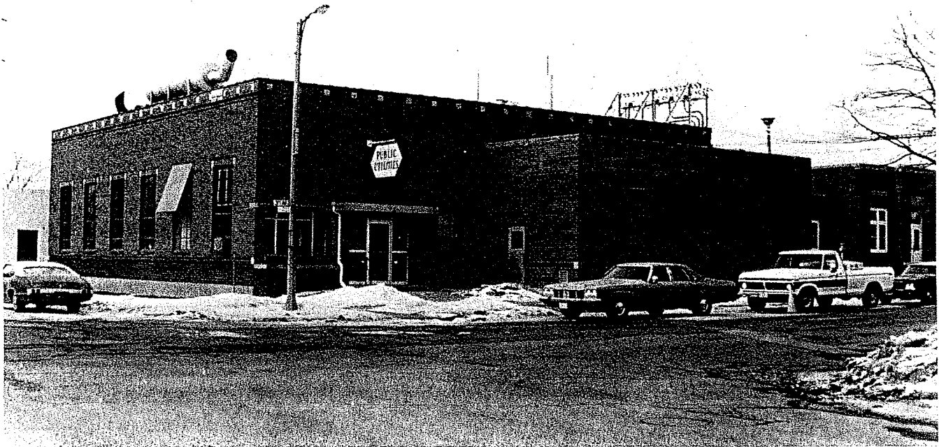
Greatly Enlarged Since the First Unit Was Built in 1931, the Municipal Utility Building is a City Landmark.
