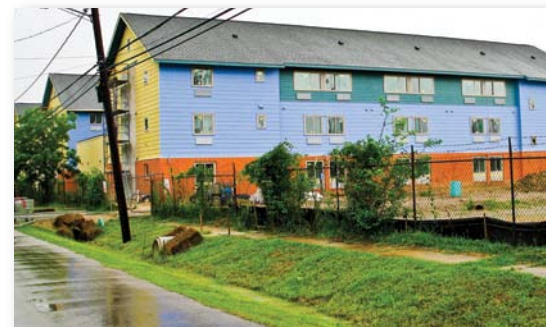
(CS Photo 23) Sakowitz Apartments under construction
