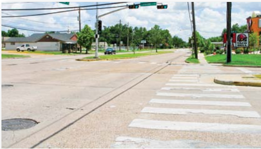
(CS Photo 18) Intersections of major thoroughfares, such as Lockwood at Cavalcade, have long pedestrian crosswalks
