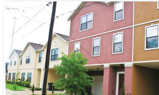
(CS Photo 22) New townhome construction in Lower French Town
