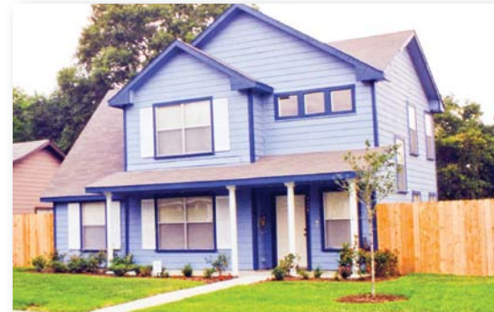
(CS Photo 21) New single family home
