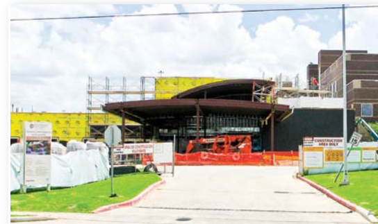
(CS photo 27) New wing of LBJ Hospital under construction
