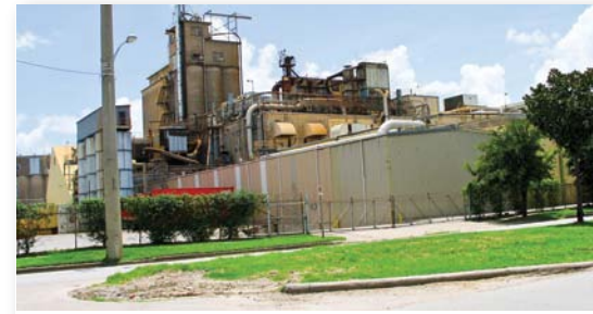
(CS Photo 3) Industrial property along Clinton Drive
