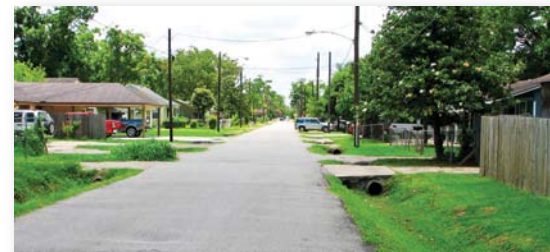
(CS Photo 17) Force Street in Denver Harbor is a local residential street that lacks sidewalks
