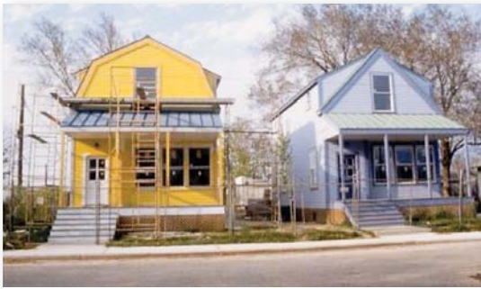
(CS Photo 1) Single family homes
