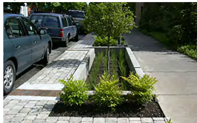
Bio-filtration in Sidewalk Area
