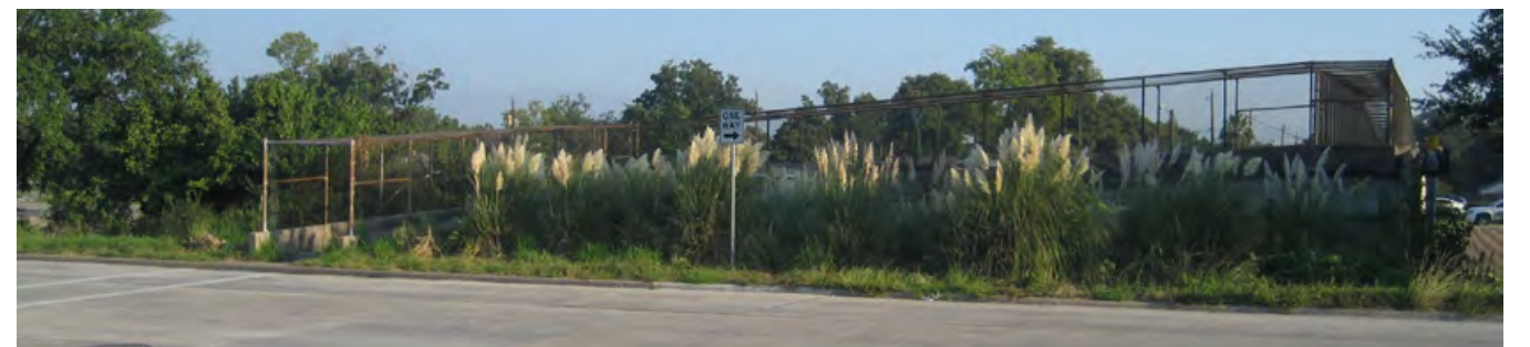
Calles Street bridge across IH=10
