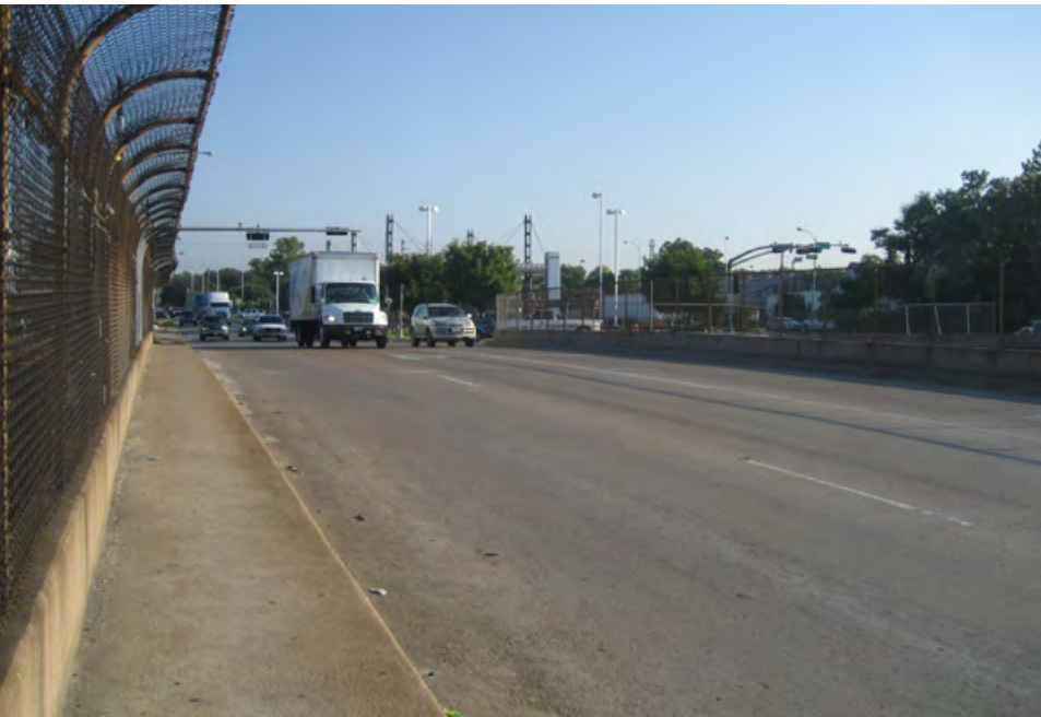
Lockwood IH-10 Overpass
