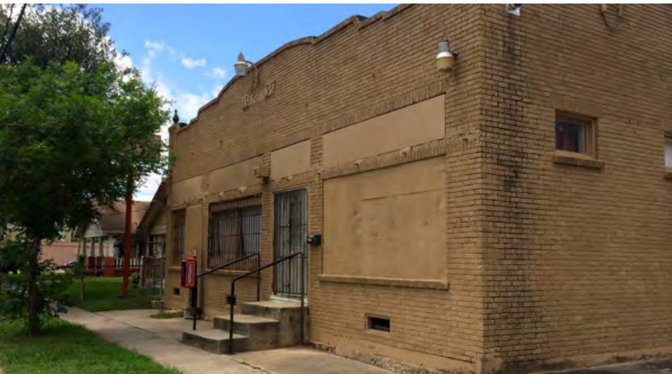
Historic building stock within the study area are attractive assets for redevelopment efforts.
