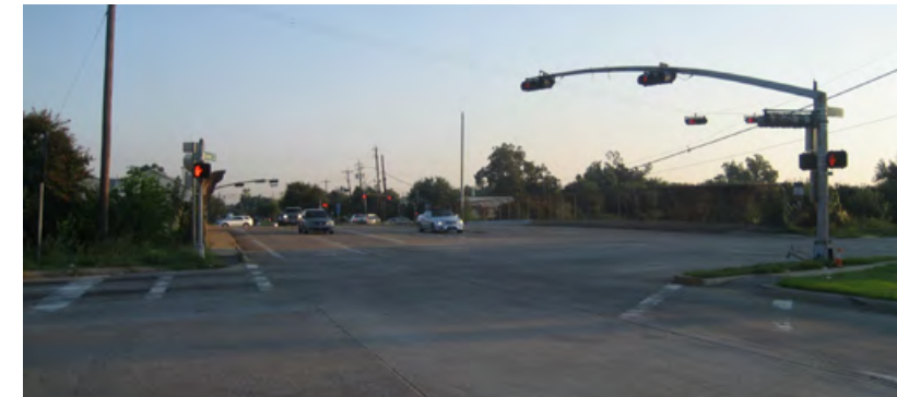
Waco IH-10 Overpass | Faded crosswalk and pavement markings
