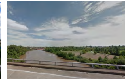
2) Hirsch Road Bridge looking east
