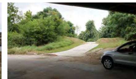
5) Under Lockwood Drive Bridge looking west to hike-and-bike trail
