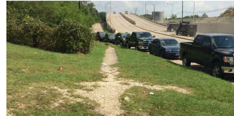
Lockwood Buffalo Bayou Bridge
