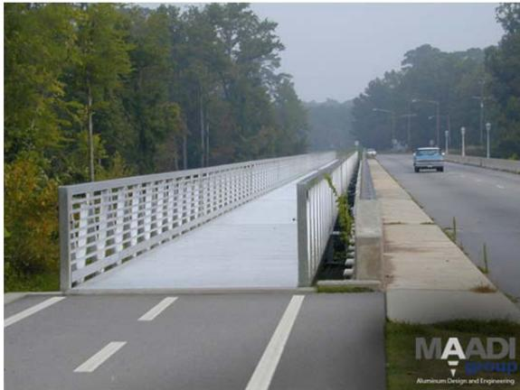
An example of a cantilevered bridge alongside existing facilities - a modular pedestrian bridge over the Tar River in Rocky Mount, North Carolina. Source: MAADI Group
