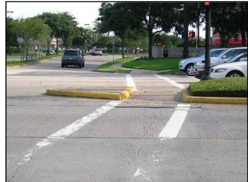
*If traffic or signal timing requires pedestrians to cross the roadway one side at a time, median refuges provide a sense of safety. Cut-throughs can be at grade, or have a ramp at either end.*
