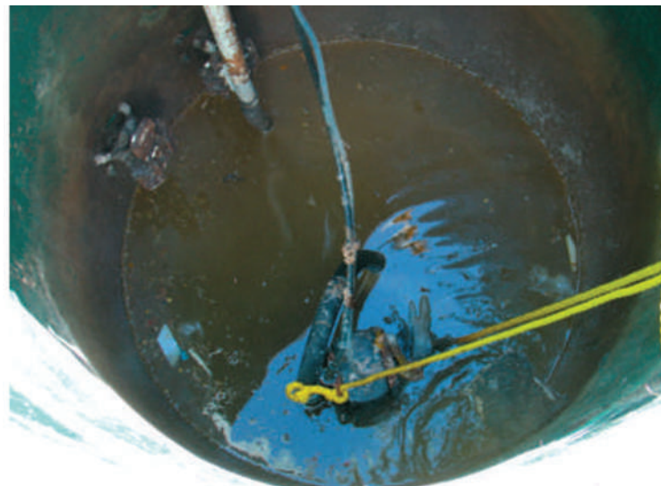
Top view showing Upgrade retrofit.
