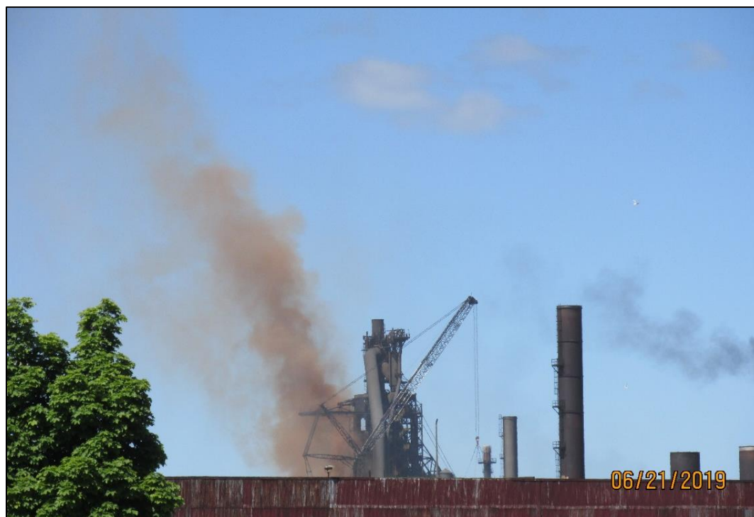
Photo 12: Heavy iron emissions from the casthouse of No.07 Blast Furnace
