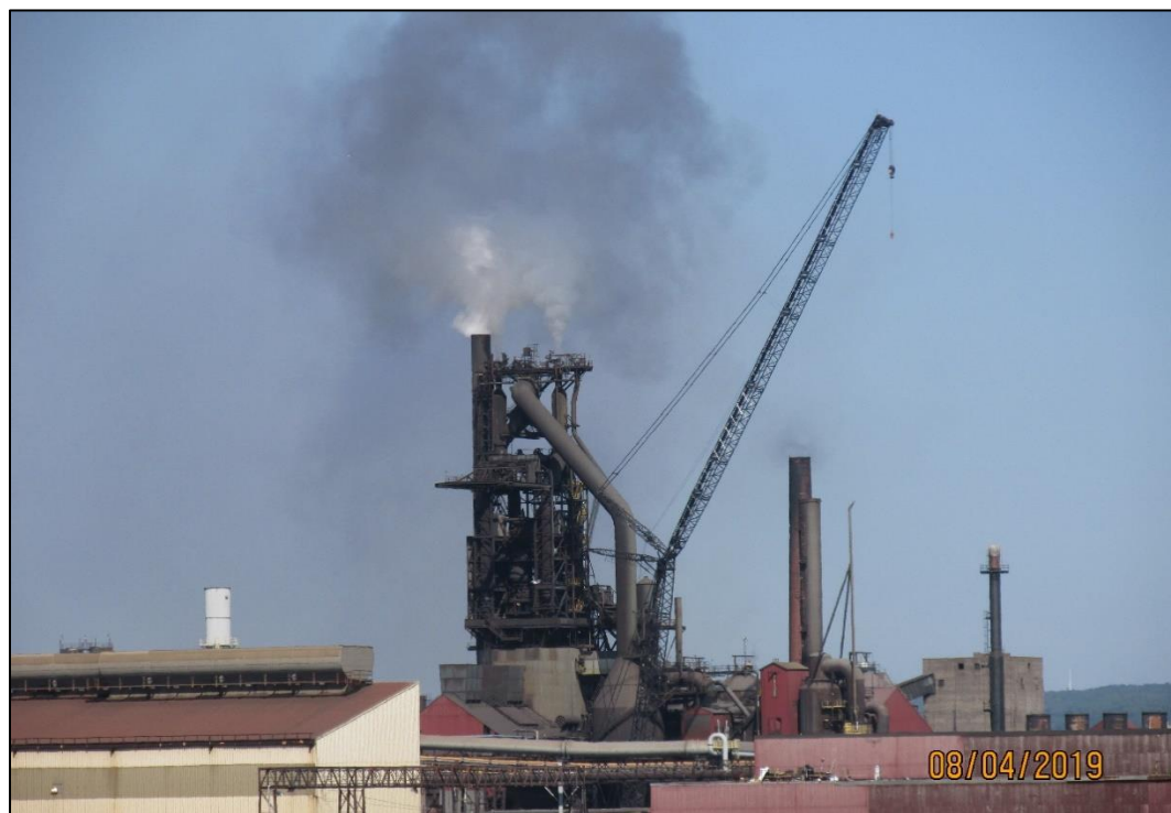
Photo 11: No. 7 Blast Furnace releasing untreated gas and particulate from dirty bleeder valves
