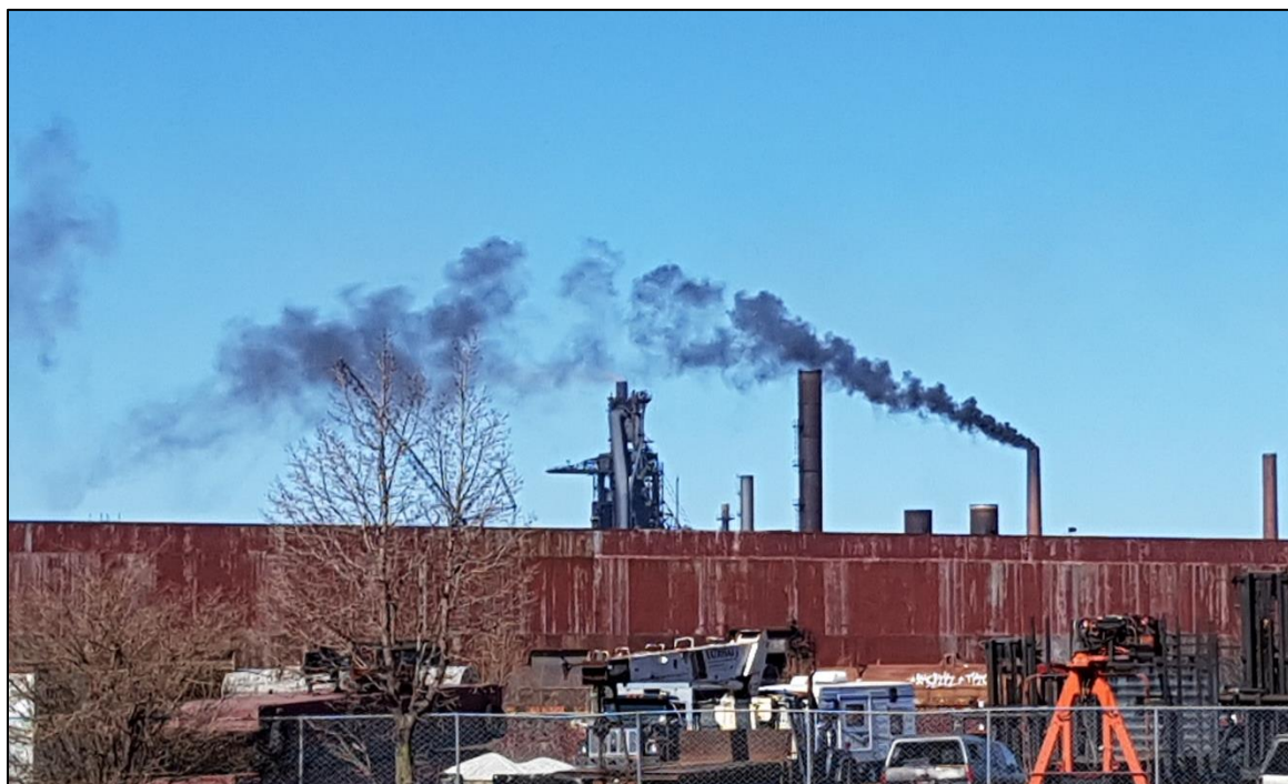
Photo 14: Very high opacity (100%) acrid stack emission from No. 7 Battery on May 07, 2019
