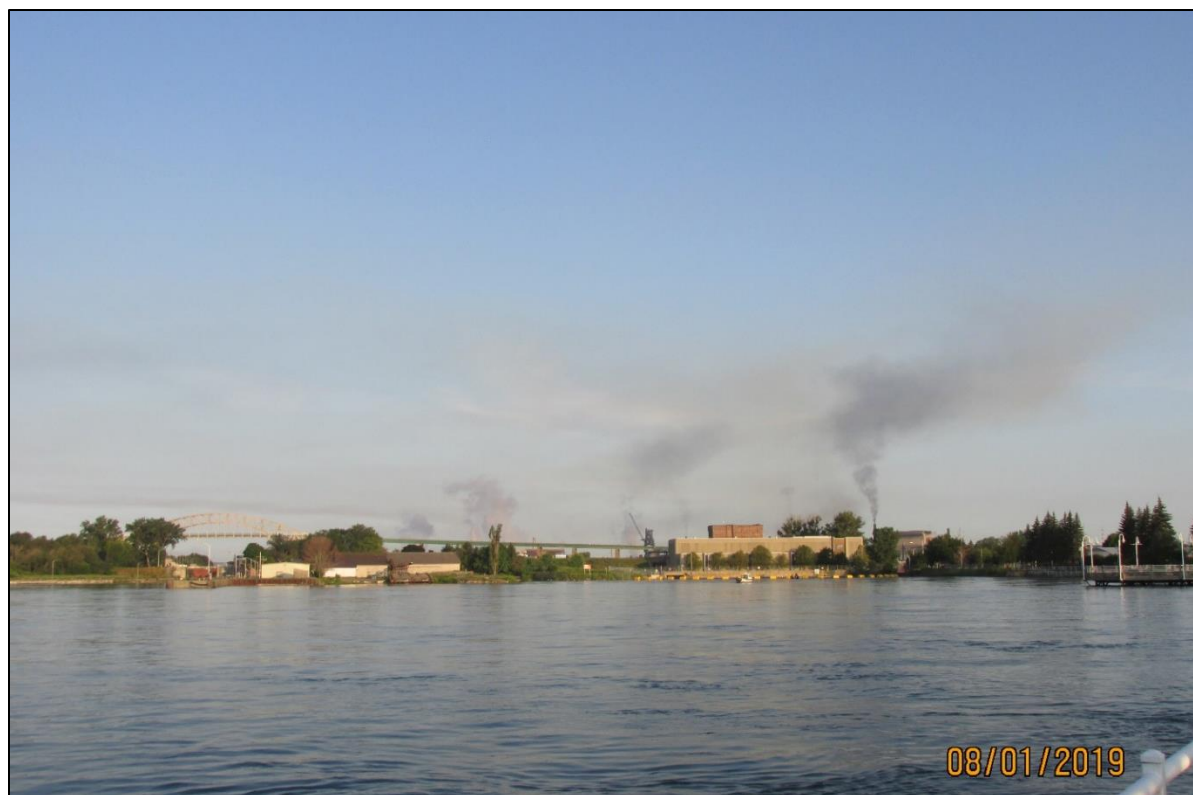
Photo 27: High opacity particulate emissions from No. 7 Battery (far right) and BOSP Plant particulate emissions
