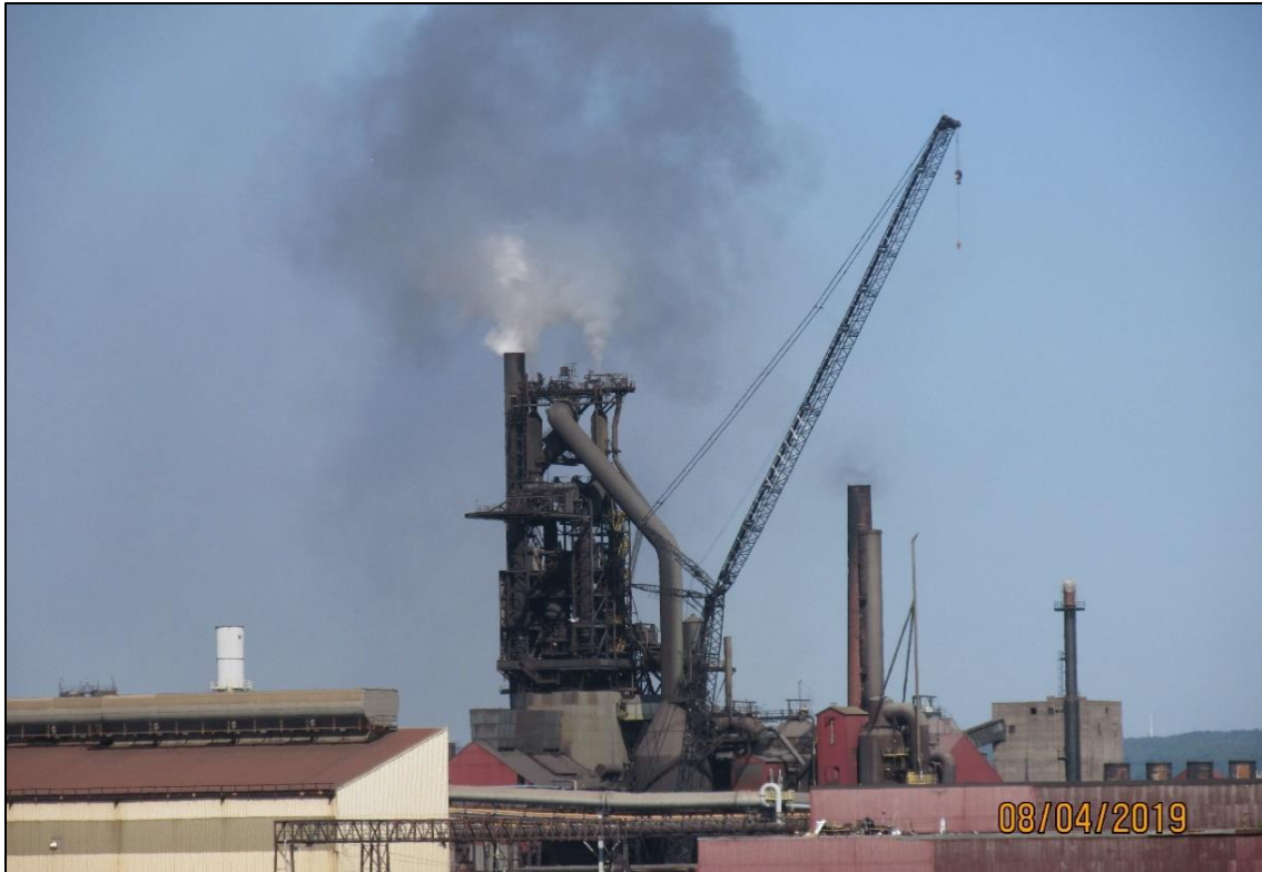
No. 7 Blast Furnace releasing untreated gas and particulate from dirty bleeder valves
