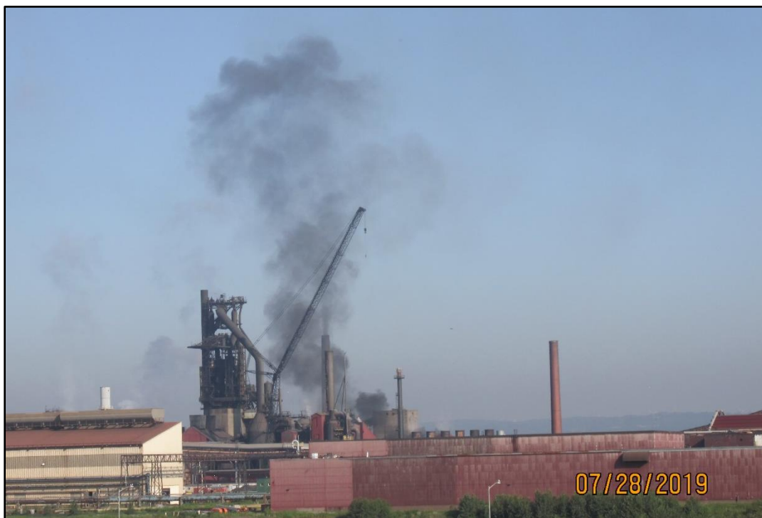
Photo 6: Heavy emissions from a failed push (emptying of coke from an oven) on No. 7 Battery
