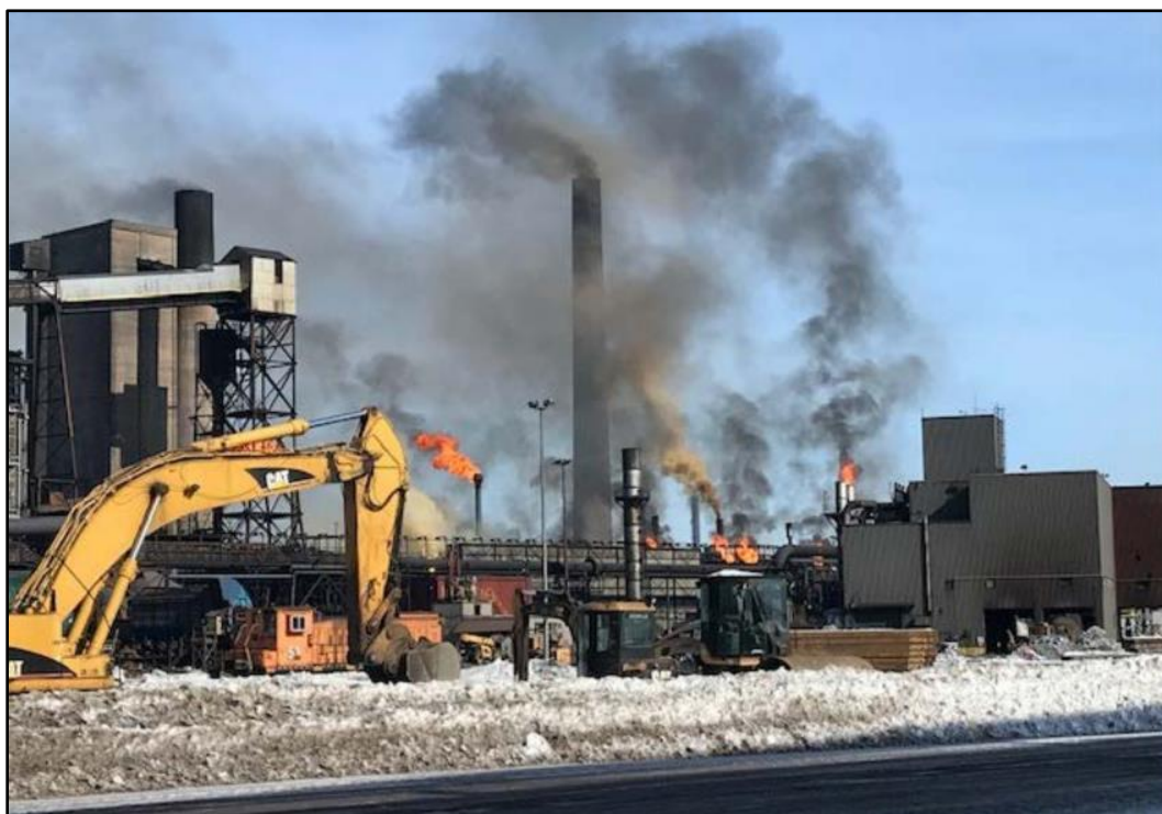
Photo 4: Flaring of coking gases from No. 8 and 9 coke oven batteries (Mar09/19).
