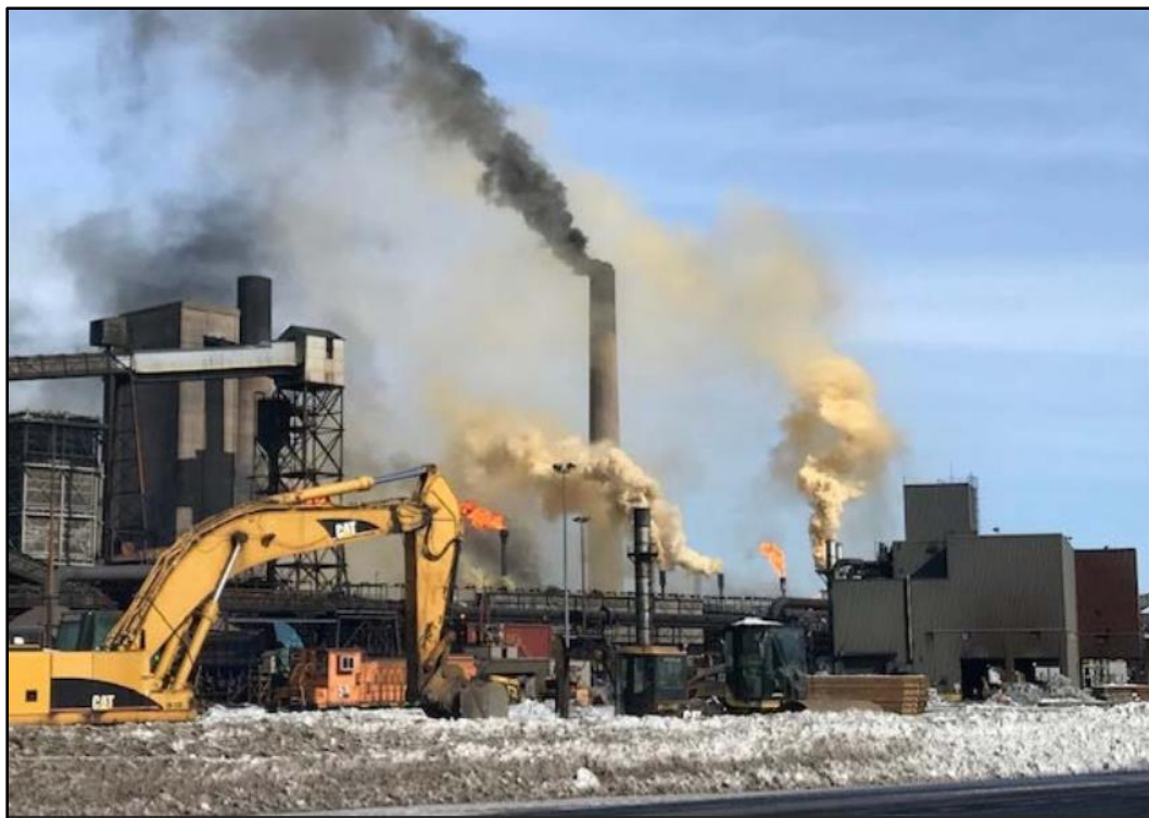
Photo 3: Raw yellow coking gases being released from No. 8 and 9 coke oven batteries (Mar09/19).
