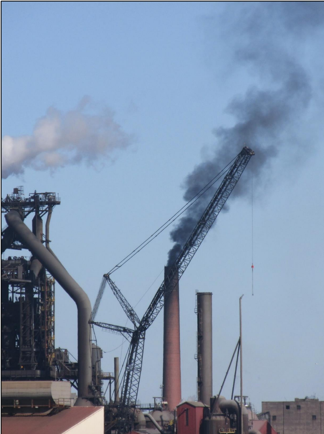
No. 7 Coke Oven Battery stack emitting particulate at 100 percent opacity on June 27, 2019
